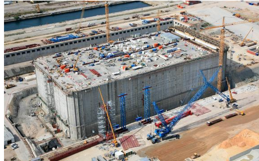
GBS end wall completed (June 2007)
